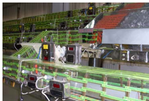
Fig. 8: Temperature sensor for test
